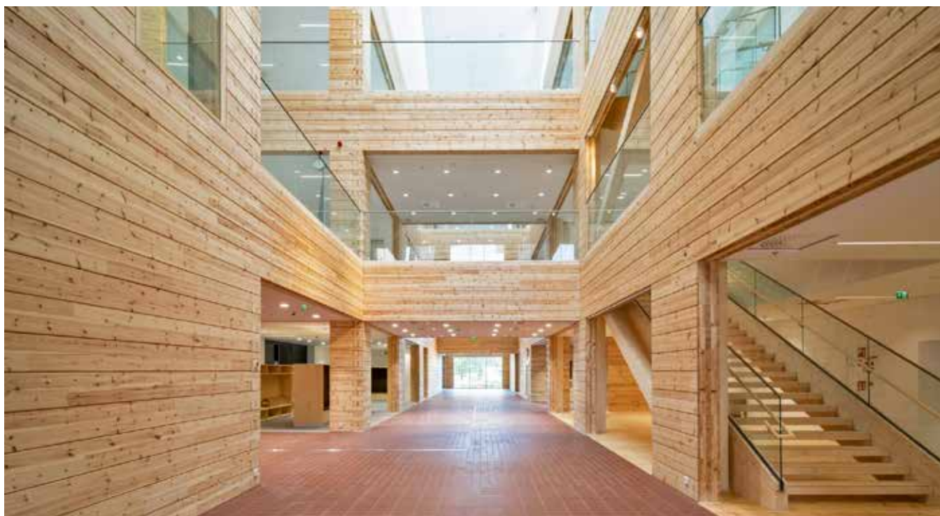
Figure 14. In Cultural Centre Monio, it has been possible to leave a lot of the log surfaces visible thanks to functional fire design. Image Kontiotuote Oy.
